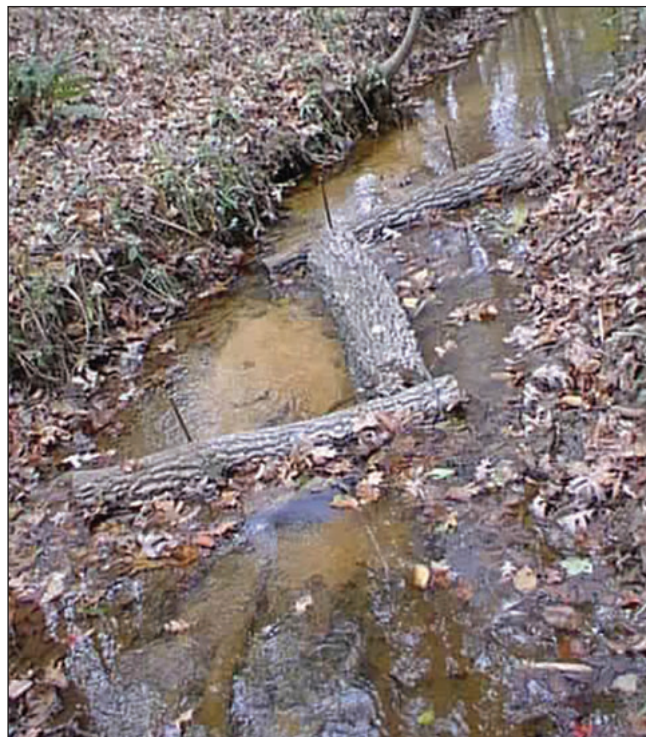
Figure 4. Artificial debris dam installed as part of a pilot-scale stream restoration project, sponsored by the US Department of Defense, Strategic Environmental Research and Development Program, at Fort Benning, GA. Restoration that promotes the storage of organic matter through the creation of debris dams has the potential to decrease downstream N loading.
