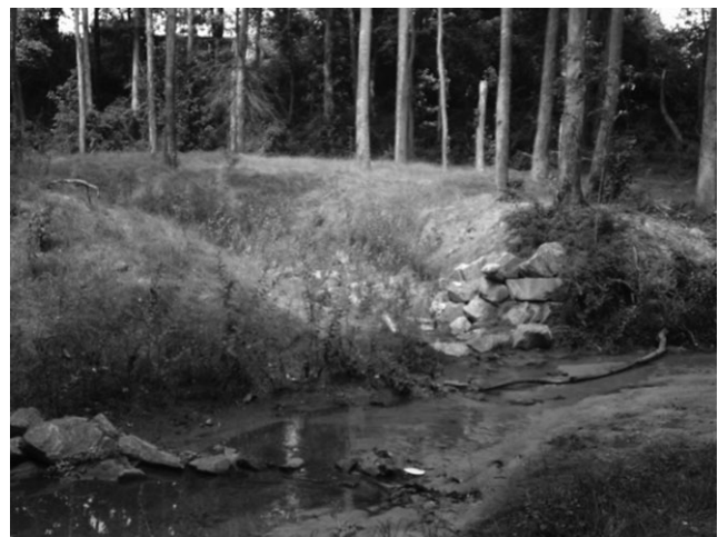
Fig. 2 Photograph showing a representative restored stream, located in northern Anne Arundel County, Maryland. Large boulders have been placed on the channel banks to prevent bank erosion and have been placed in the channel to prevent channel incision.
